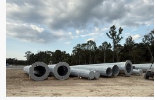
Delivery of T-line poles
