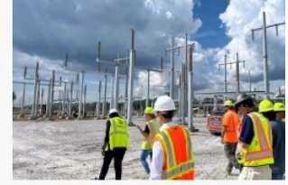
Onsite coordination with Entergy in preparation center buildout
