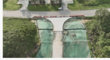
Construction of Entergy permanent access road
