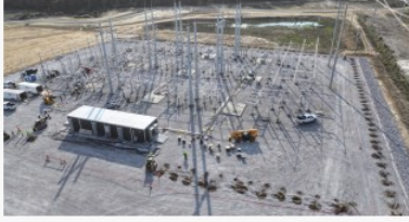
Construction of switchyard
