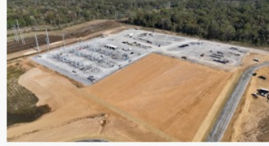
Grading and preparation for substation construction
