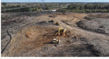
Clearing and rough grading of data center footprint
