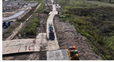
Preparation for installation of transmission line conductors
